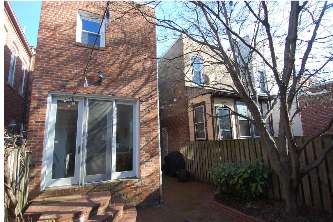
3 Rear Elevation looking Southeast A-3 N.T.S.
